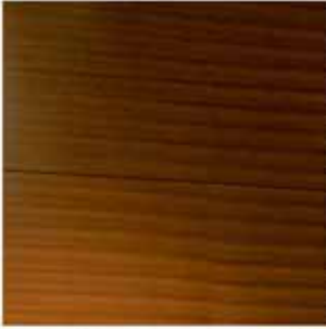
EXISTING WOOD PANELS
